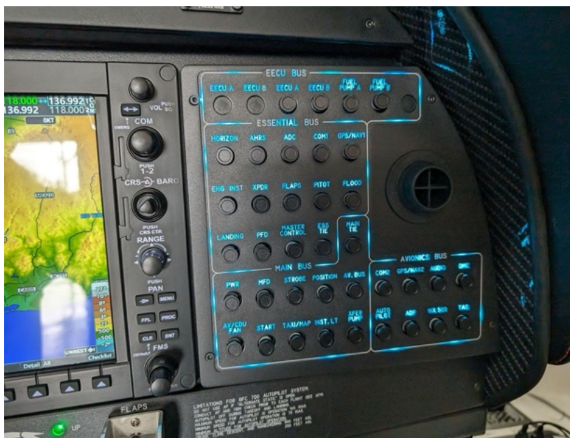
Image 6. View of circuit breaker panel
